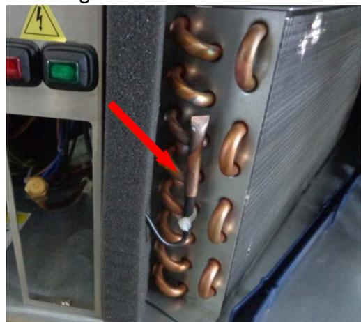
The condenser temperature sensor probe is located in the condenser, which detects the condenser temperature variations and transmits electronic signals to PC board.
