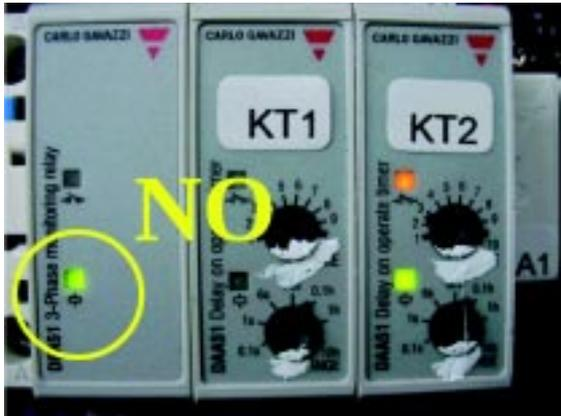
6. Correct wiring is shown by both LEDs Green and Orange steady ON together.
